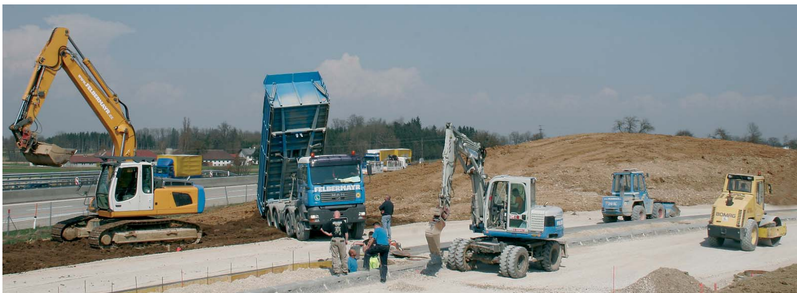
Around 20,000 cubic metres of fill was needed for the road and landscaping, including the relocation of 2,500 cubic metres of humus from an ecologically significant area of grassland (to the right of the picture).
