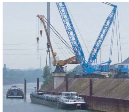
The transformer was changed over in the Felbermayr heavy goods port in Krefeld.
