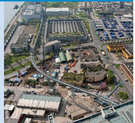
The fuel from the treatment plant is transported to the power station via a 460 metre long conveyor.
