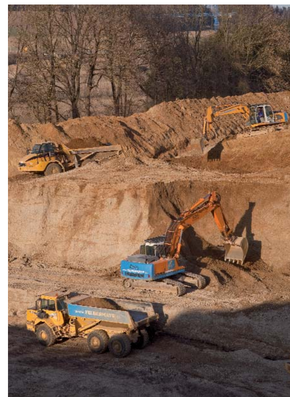
The material needed to build the embankment came from close to the site. After project completion, the 26,000 m 2 area will be carefully renatured.
