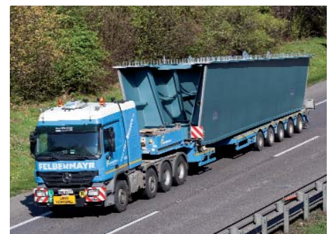
The bridge elements were transported to the site »just in time«. They were manufactured by NCA Container- und Anlagenbau GmbH in St Paul, Lavanttal
