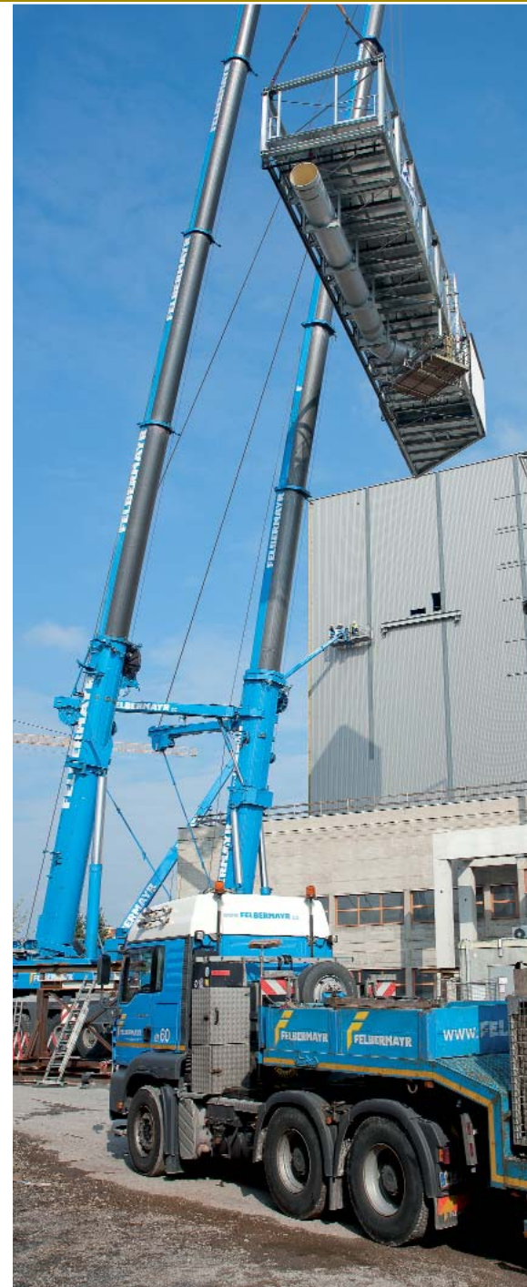
The lifting LTM 1500 was fitted with a Y-anchor and 160 tonnes of ballast. Only 72 tonnes were needed for the back-up crane.
