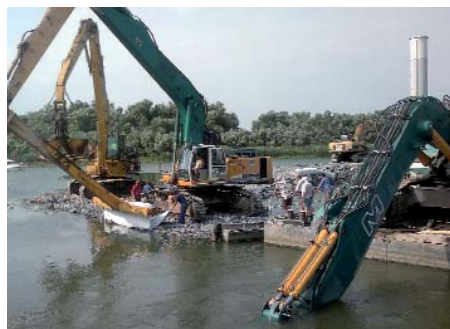
55,000 square metres of geotextile fibre layers were installed for the protective measures.
