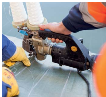
After filling the air mattresses with concrete, the openings were sealed.
