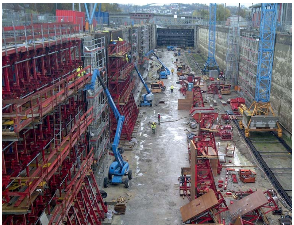
For concreting the facing formwork on both lock chambers more than 6000 square metres of formwork had to be built.
