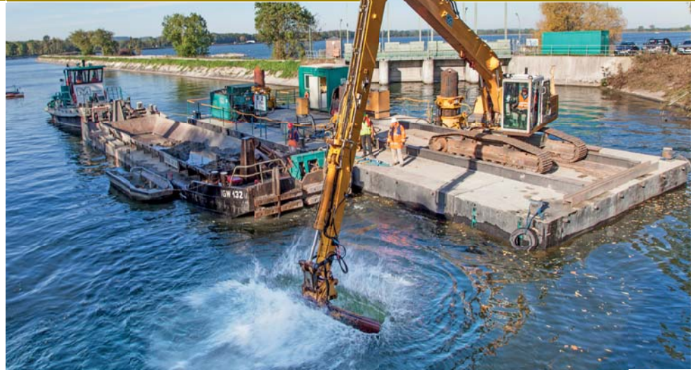
Long-arm excavators were used to profile the canal bed which was up to seven metres deep.
