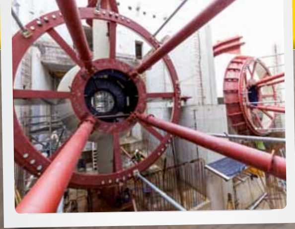
The ANDRITZ Hydro turbines were later fitted to these two "mounting spiders".
