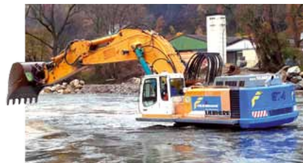
Among the equipment used to move over 300,000 cubic metres of material was an 87-ton excavator.
