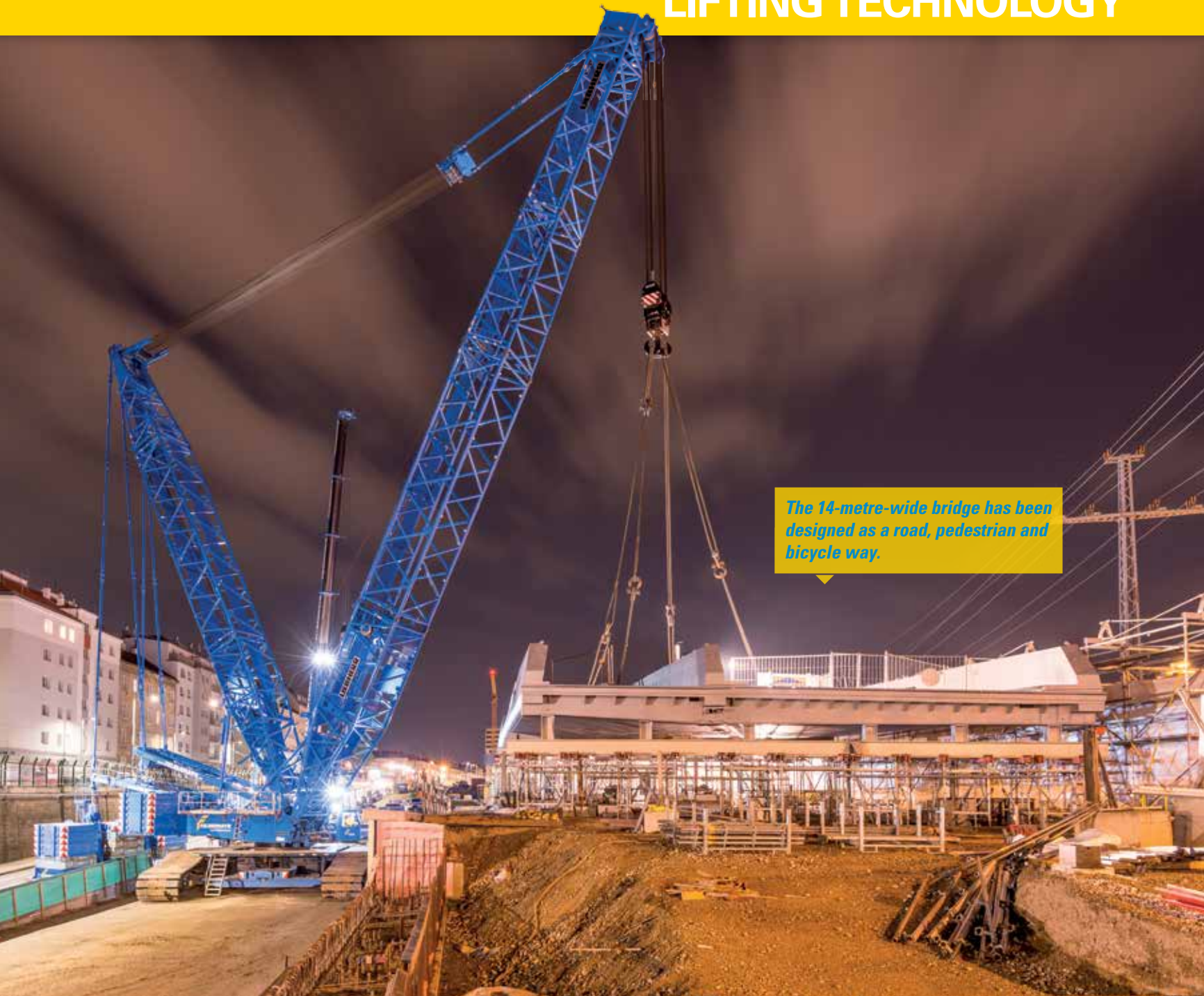
The crawler crane was equipped with 270 tonnes of suspended ballast.
