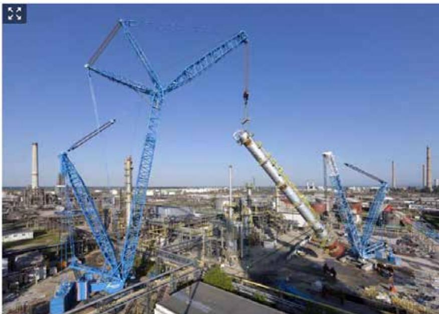
**Felbermayr's Liebherr LR 11000 and a LR 1750 crawler cranes work in tandem to lift the column**
