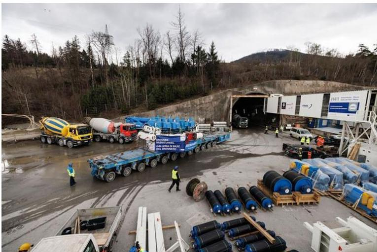
A great deal of logistical effort was required to drive the components - weighing up to 270 tonnes - through the narrow tunnel to the assembly caverns.
