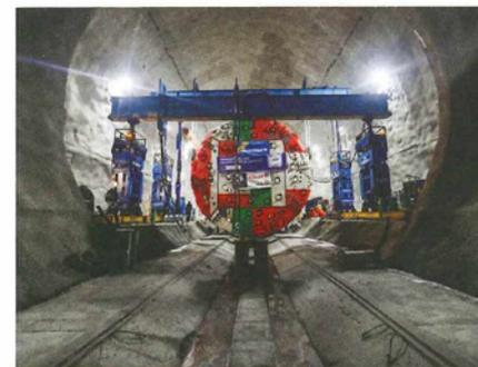
After the tricky transport Felbermayr also assembled the TBM. Here the cutter head has been tilted up to vertical with the help of telescopic hydraulic lifting gantries
