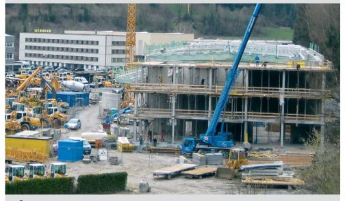
n office building of more than 1,000 m² was constructed by the Felbermayr Construction department for the Liebherr works in Bischofshofen. The scope of the commission for the frame construction building ranged from installing the floor slab, various formwork tasks for in-situ concrete columns and floor units, to assembly of the facade elements. The concrete structure for the three-storey office building was completed in May. A total of 600 cubic metres of concrete was used.
