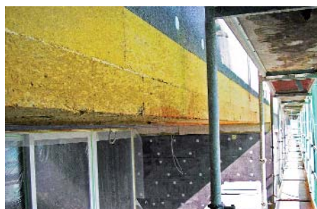
The mineral wool fire protection strip prevents the spread of fire and stops the dangerous dripping of molten insulation system components.
