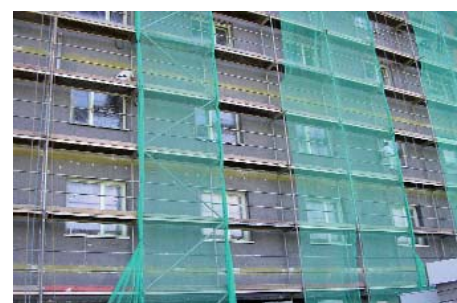
Lamdapor of 22 and 28 centimetre thickness was used for the insulation of the upper storeys, with reinforcement from Capatect 190 adhesive and filler compounds, finished with Capatect CarboPor textured finish, grain size 30.
