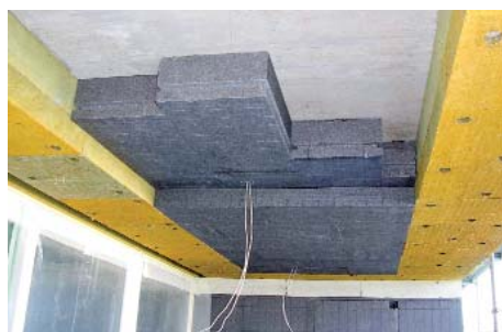
The two-layer installation of the insulation requires a high level of expertise with relation to the adhesive, insulation material and plugging.
