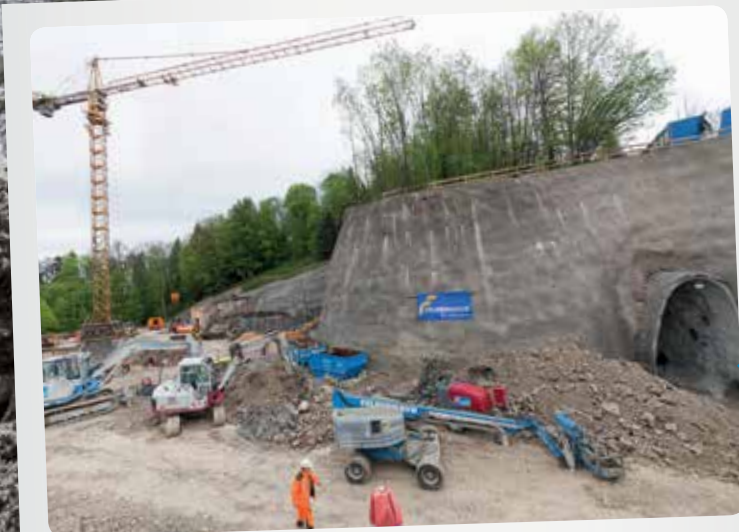
The scope of the order included the temporary construction pit system and the construction of a 50-metre tunnel.
