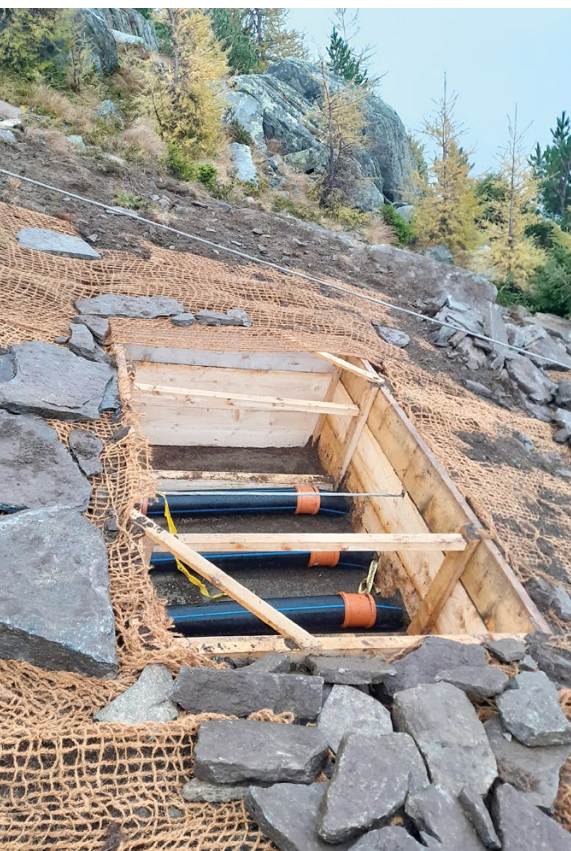
The cable is fixed at a total of 14 fixed concrete points after the cable pull in the steep section.
