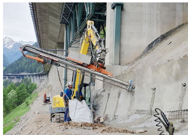
Nailed shotcrete walls secure the steep slope along the path. To do this, soil nails are inserted using drilling equipment.
