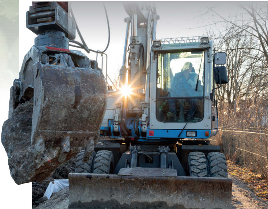
An excavator positioned the armour stones in transportable chunks for the crane to collect.
