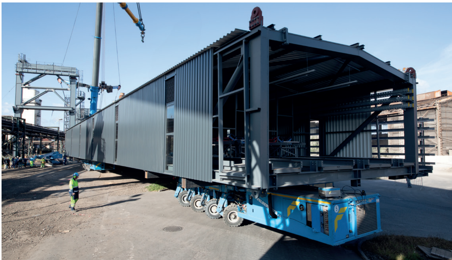
The SPMT was used to lift the pre-assembled segments of the conveyor belt bridge into position under the cranes. With lengths of up to 62 metres, the seven elements weighed up to 180 tonnes each.
