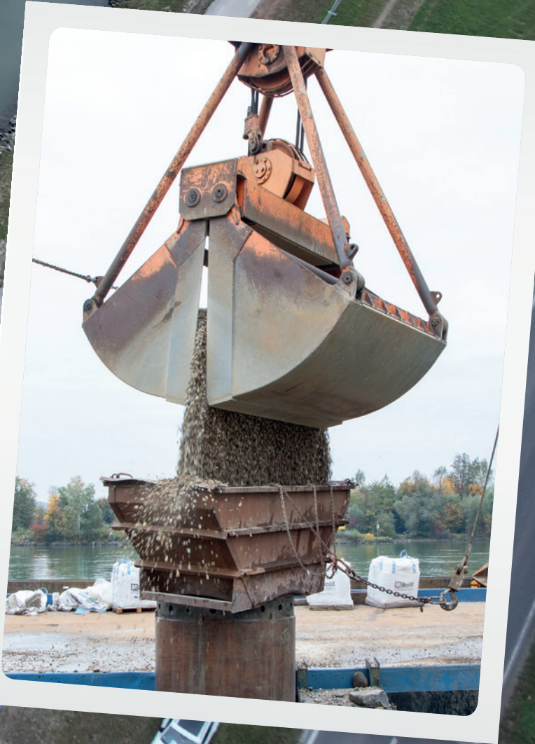
In all, 1,200 tonnes of gravel was used to backfill the pile moorings.
